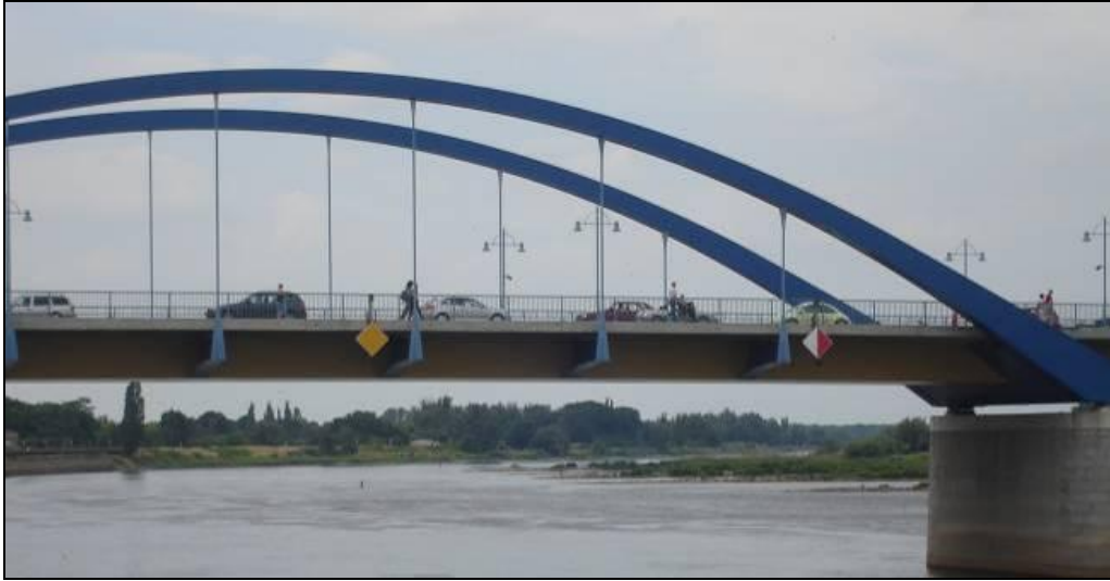
Figure 5.11 The Bridge Connecting Słubice and Frankfurt-Oder
